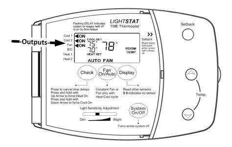
You can use the output indicators to help troubleshoot your HVAC system. If the **Cool 1** and **Cool 2** output indicators are displayed, you should feel cool air coming from the HVAC system. If a Supply Air Sensor is installed, you should read the temperature of the cool air coming from the unit.
